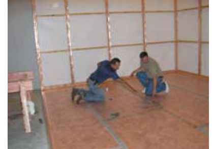
Monolithic Copper Flooring
