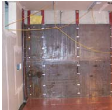
Steel Plate Shielding
